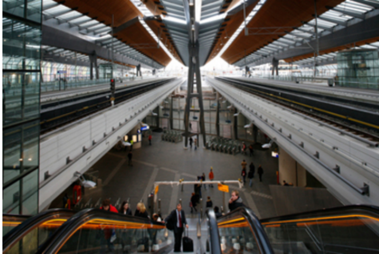
1 Bijlmer Arena Station concourse and platforms Source: www.jaaphuisman.nl
