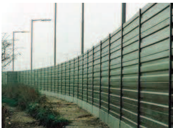
Acoustic Barrier against road noise, shrubs trees and greenery will visually 'soften' the dwelling side.
