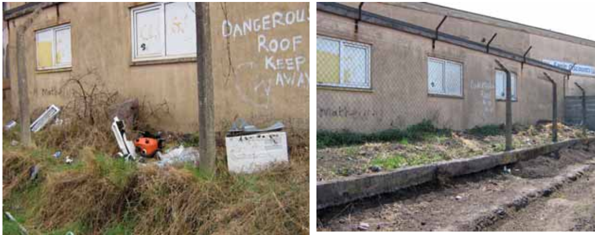
Fly Tipping Improvements in rear lane Henshaw Street
