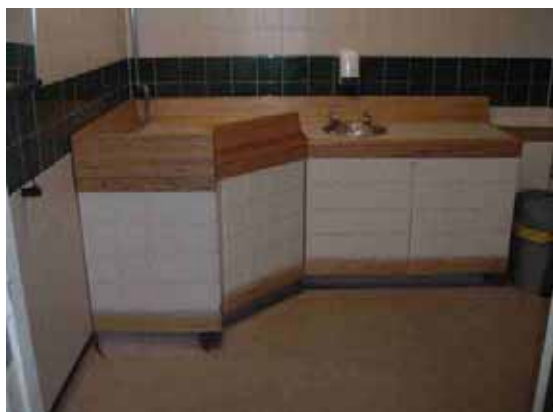
Figure 13 – Accessible toilet and baby change facility.
