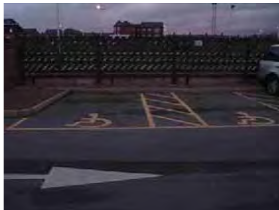
Figure 2 – Accessible parking bays.
