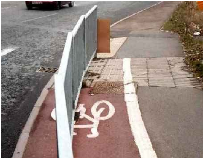
Figure 1: Half-width bicycle facility
